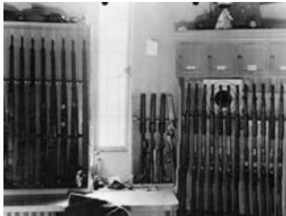
San Quentin Prison guns. Security Pacific National Bank Photo Collection, Los Angeles Public Library.
