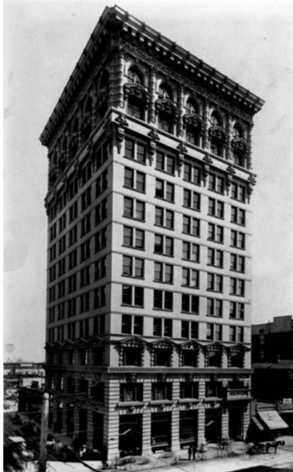
FORMERLY BRALY BLOCK, CALIFORNIA RESERVE BUILDING 408 SO. SPRING STREET (JOHN PARKINSON, 1904)
