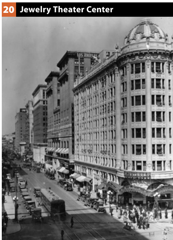
ORIGINALLY PANTAGES THEATRE BUILDING; WARNER BROS. DOWNTOWN THEATRE 401 W. 7TH STREET (B. MARCUS PRITECA, 1920)
