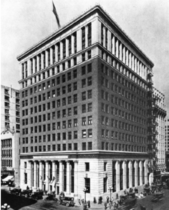
505 WEST SEVENTH ST. (MORGAN, WALLS & MORGAN, 1922)
