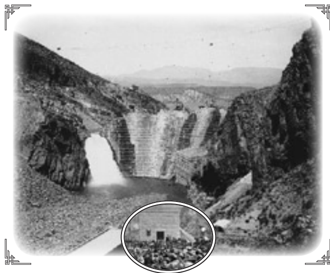
ROOSEVELT DAM, located on the Salt River, currently supplies much of metropolitan Phoenix, Arizona, with both water and hydroelectric power, and is often involved in litigation and negotiations with competing water interests. Inset photo, bottom: Theodore Roosevelt speaking in 1911 at the dedication of Roosevelt Dam, the first major project to be completed under the U.S. Reclamation Act of 1902.
